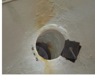
Temporary repairs on hull performed by diver on another vessel
