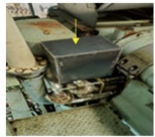
Guard fabricated to cover fuel system buffer (damping) tank
