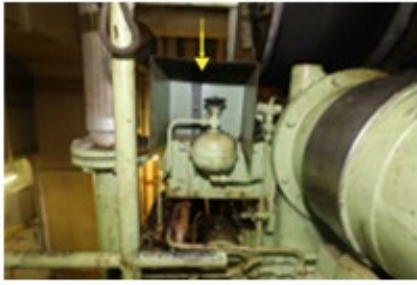
Spray shield around the pressure damper on auxiliary engine
